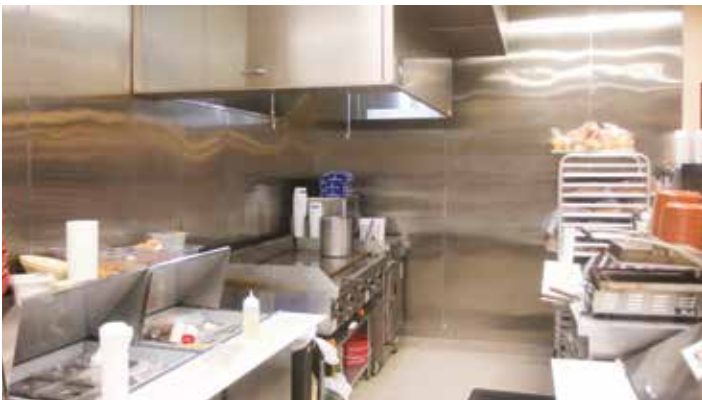
Cook stove with stainless steel hood with ansul system and prep area.
